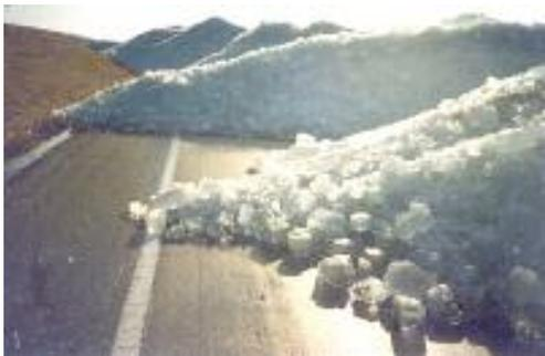
Fig. 4. Ice drift on the IJsselmeer Dam
