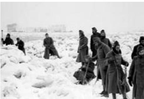
Fig. 7. Men trying to reduce the ice load on a dike
