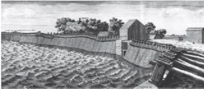
Fig. 10. Wooden piles protecting the Diemer sea dike near Amsterdam (N. Listingh, 1702)
