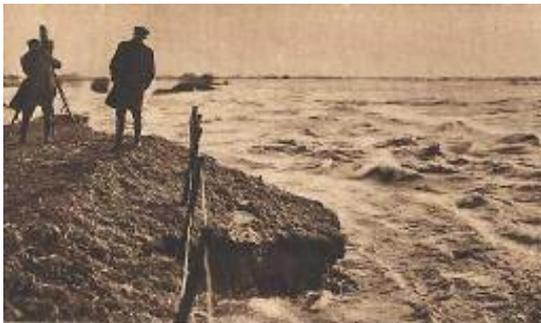
Fig. 2. Overflow of dike along the river Maas after heavy rain, Nederasselt, 8 January, 1925
